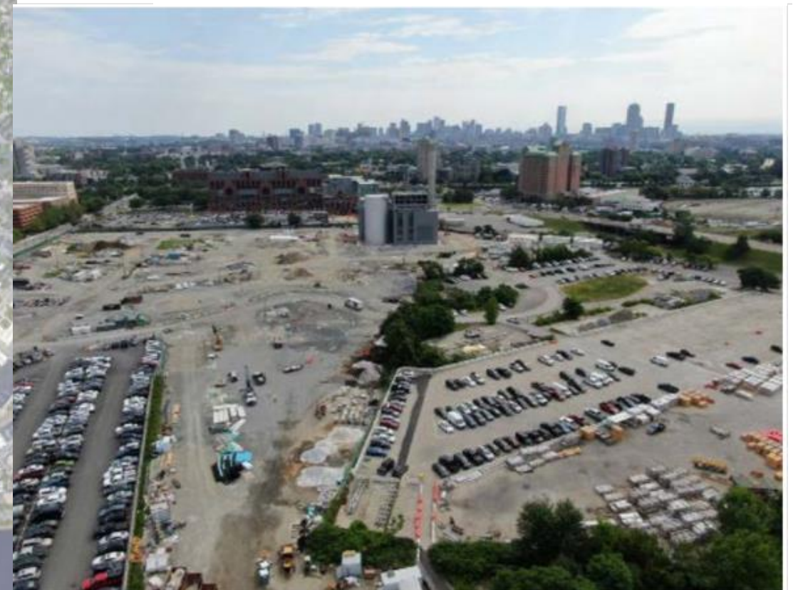
Aerial View of Current Site Conditions (2020)
