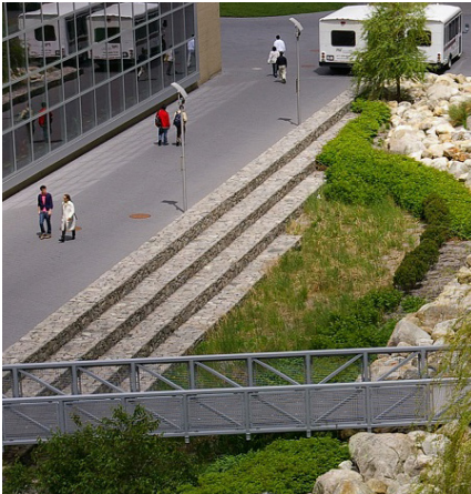
A .14 acre bioretention basin provides infrastructural and ecological benefits to the project.
