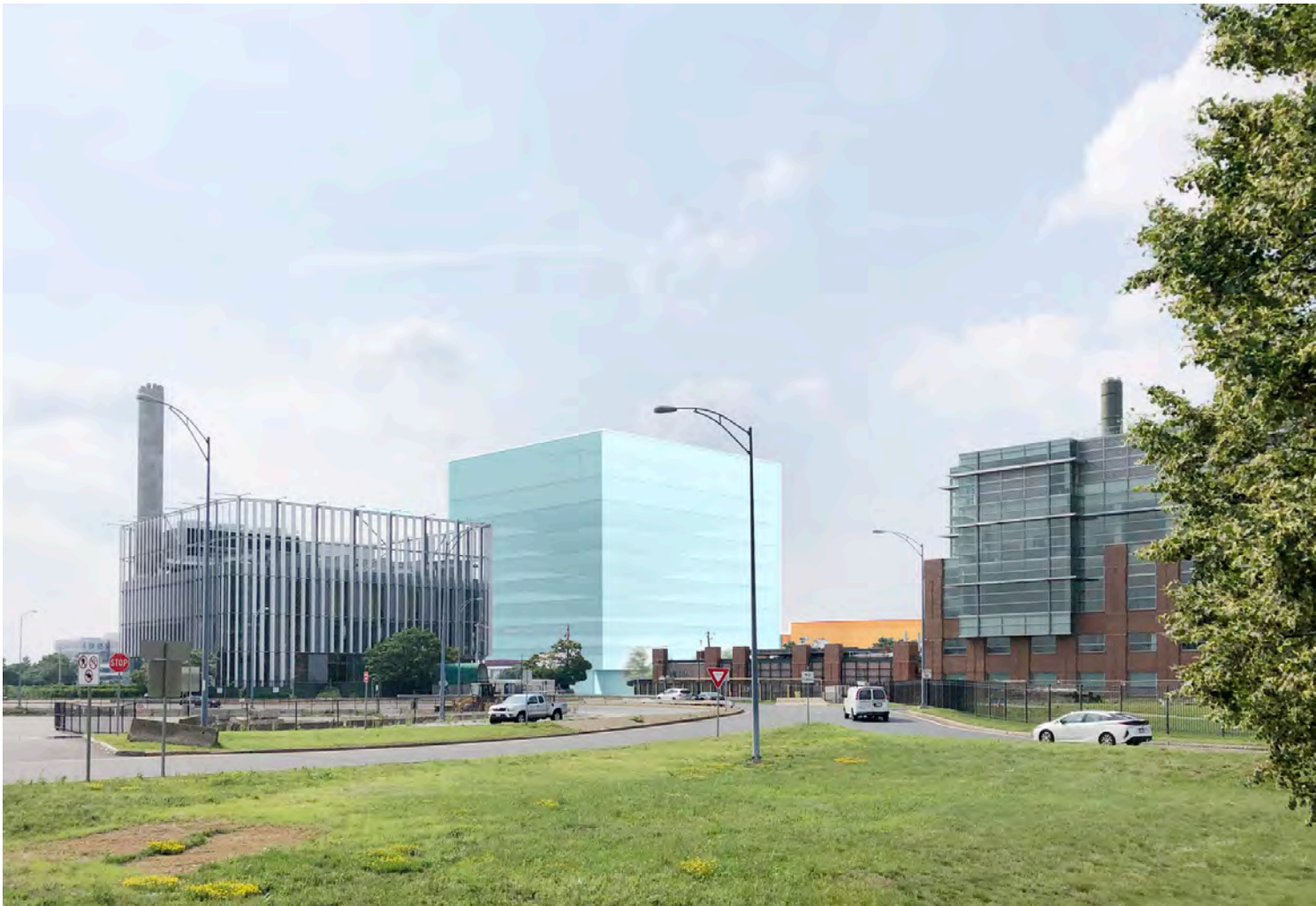
PHASE A CONDITION
