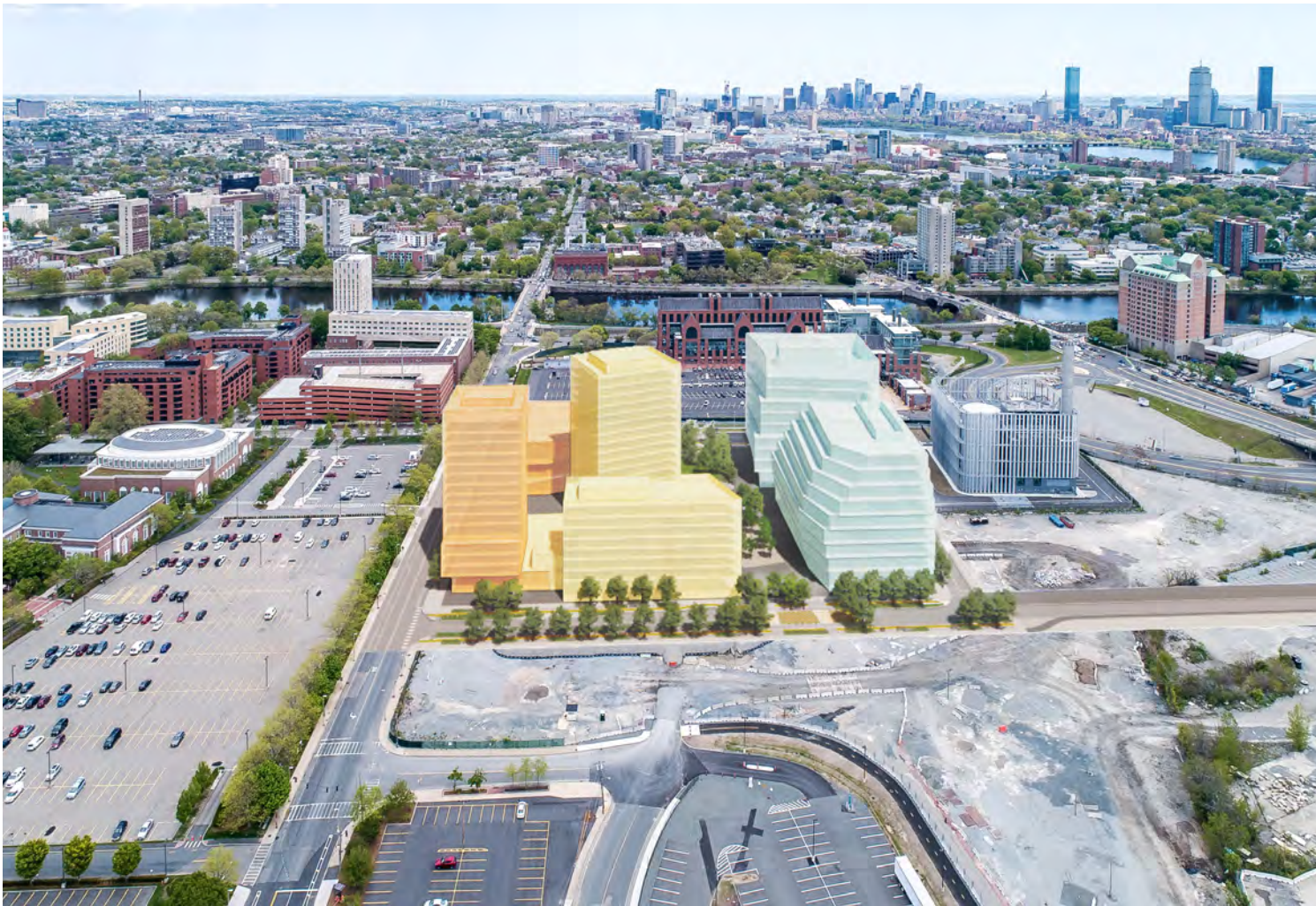
PHASE A CONDITION
