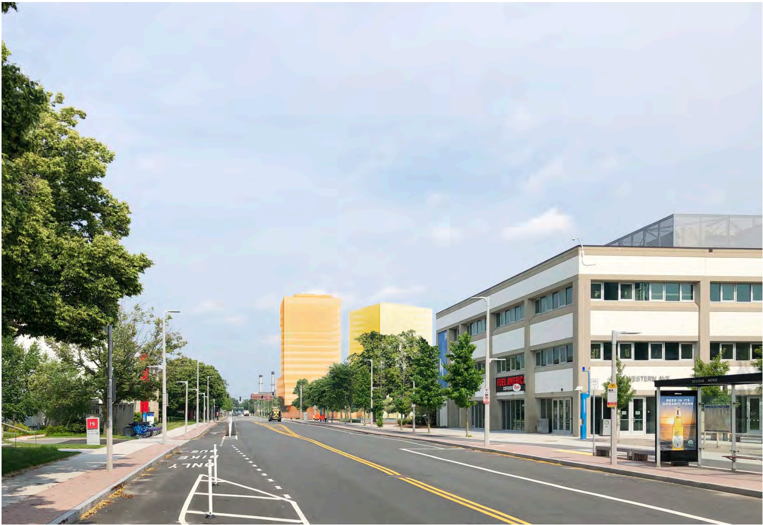
PHASE A CONDITION
