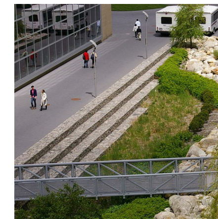
A .14 acre bioretention basin provides infrastructural and ecological benefits to the project.
