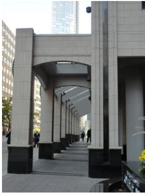
Building façade set back using colonnade
